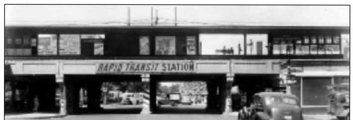
Morse Avenue “L” Station, n.d.
