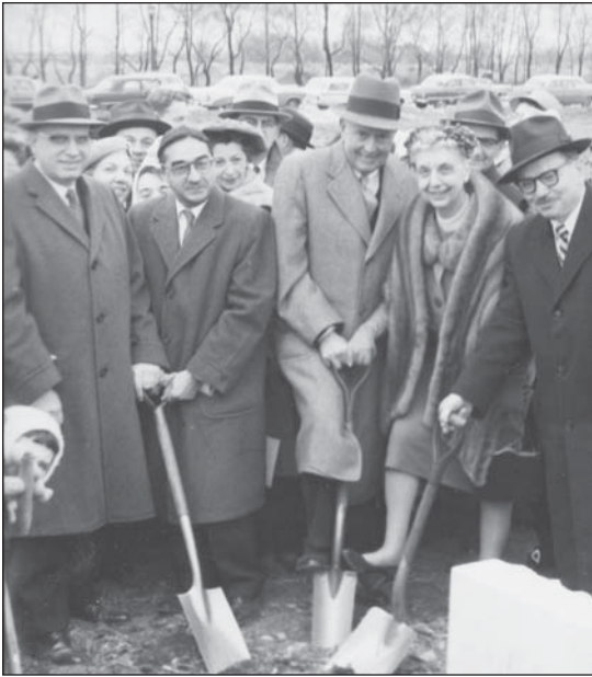
Groundbreaking for the new building, April 26, 1959. From left: Frank Kaplan, Barney Gordon, Evanston Mayor Kimbark, U.S. Rep. Church, and Rabbi Zaiman. Chicago Jewish Archives, Spertus Institute.
