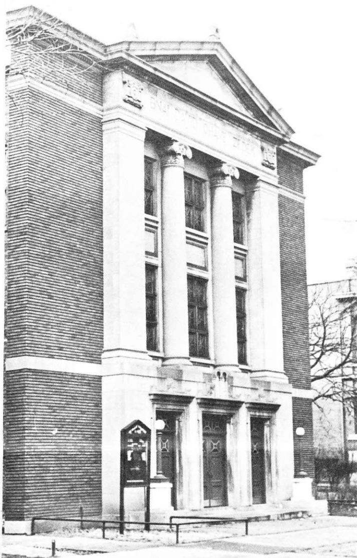
Humboldt Boulevard Temple Exterior View in 1952
